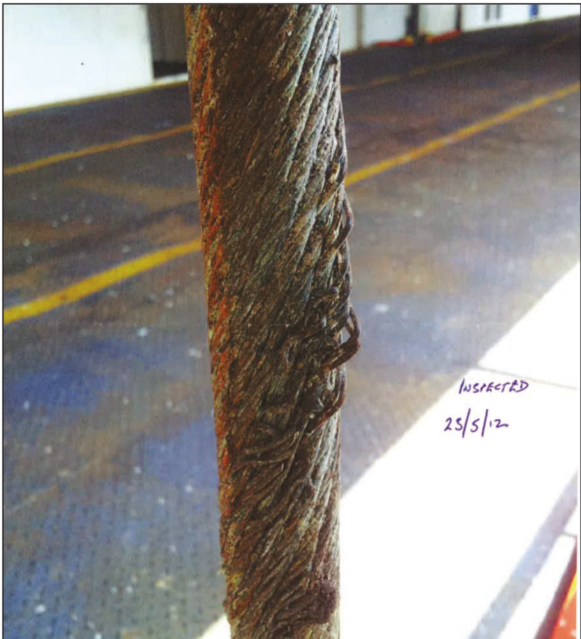
Figure 18: Photograph taken of a damaged mezzanine deck lifting rope by crew on board St Helen following an inspection carried out on 23 May 2012
