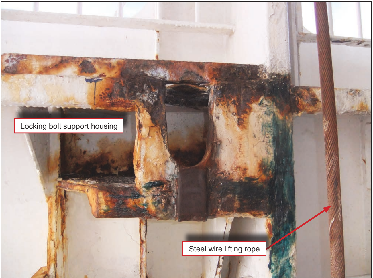
Figure 9: Mezzanine deck retractable locking bolts
