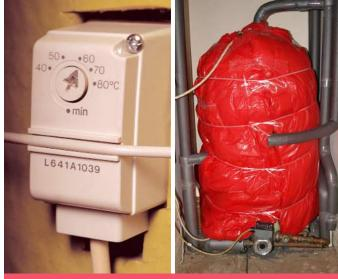
A cylinder thermostat (left) will stop you wasting money on overheating your water, while to save more on water heating, make sure you get your hot water cylinder and pipes insulated too
